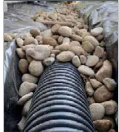
French drain around basement
