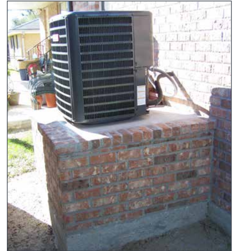
Elevated exterior HVAC equipment
