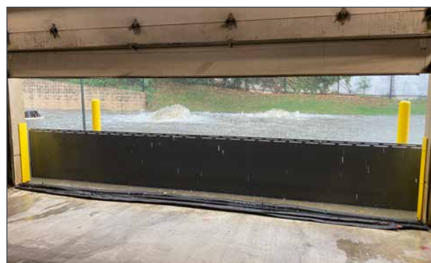
Passive flood gate at entrance to parking garage SOURCE: CITY OF ALEXANDRIA
